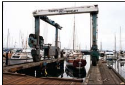
The existing 70-ton Travelift pier is 40 years old.
